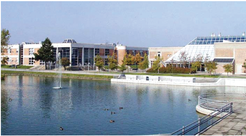
Picture 1.5 International Center for Innovation located at Aalborg University, Fibigerstraede 16, DK-9220, Aalborg, Denmark.
