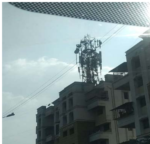
Figure 10-2 SIX STORY BUILDING SITE AT HOCKEY STADIUM.
