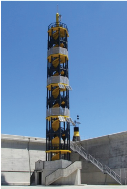
Figure 7.12 Valencia lighthouse (Spain).
