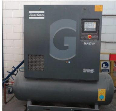
Figure 7.29 Detail of the main compressor that supplies compressed air to the resin injection system.
