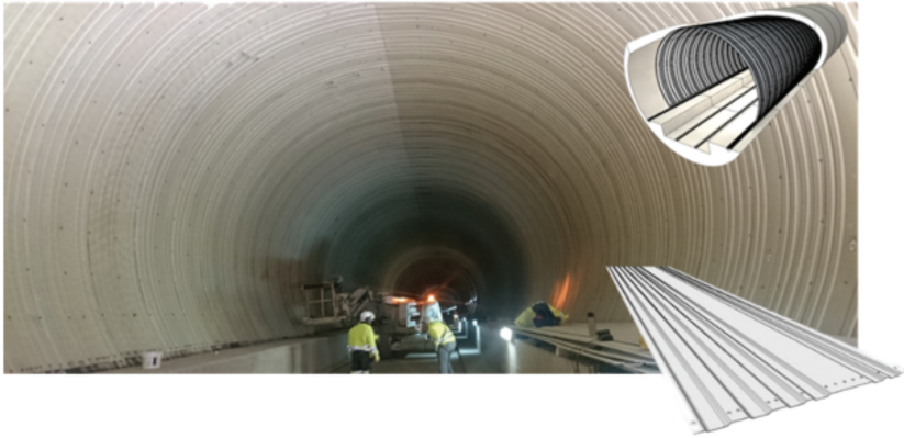
Figure 7.11 Waterproofing the Pajares tunnel in Asturias, Spain.
