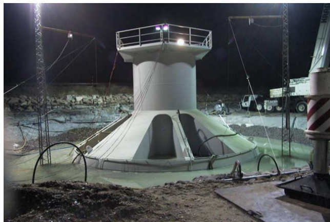
Fig. 3. Bucket foundation after installation in Nov. 2002
