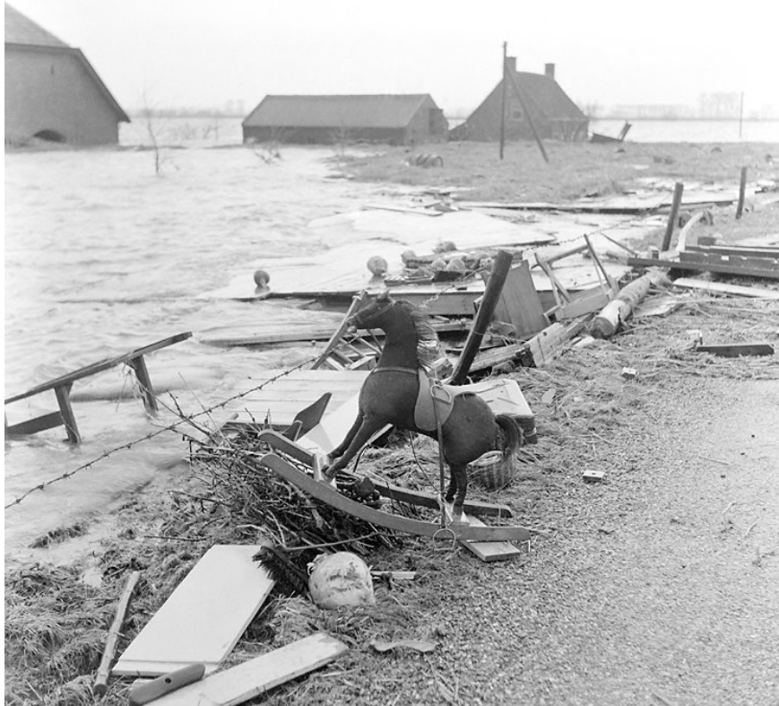
Damage after flood in the Netherlands, 1953 (Art Klein, Nederlands Fotoarchief)
