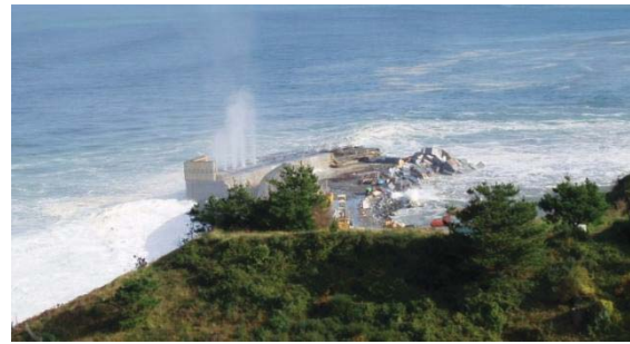
Figure 1: Mutriku plant in construction. The picture shows columns of water flowing through the holes of the power take-off system.
