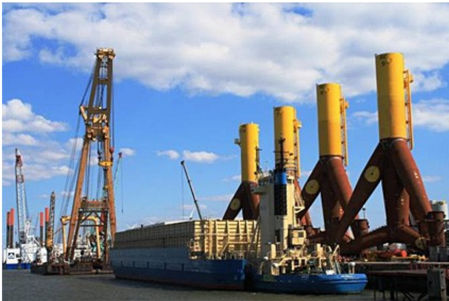
Figure 1.9 Tripod foundation for Alpha Ventus OWF (from www.aveva-wind.com )
