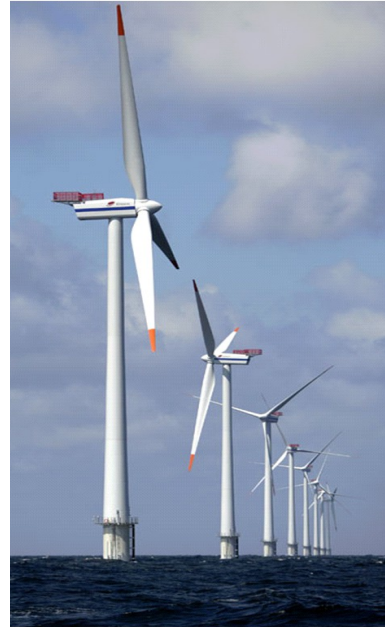
Figure 2.8 Wind turbines at Horns Rev ( www.hornsrev.dk )
