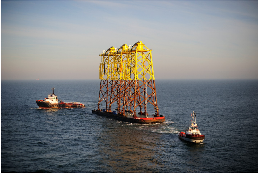
Figure 1.10 Jacket foundation for Alpha Ventus OWF (from www.lorc.e-kvator.com )
