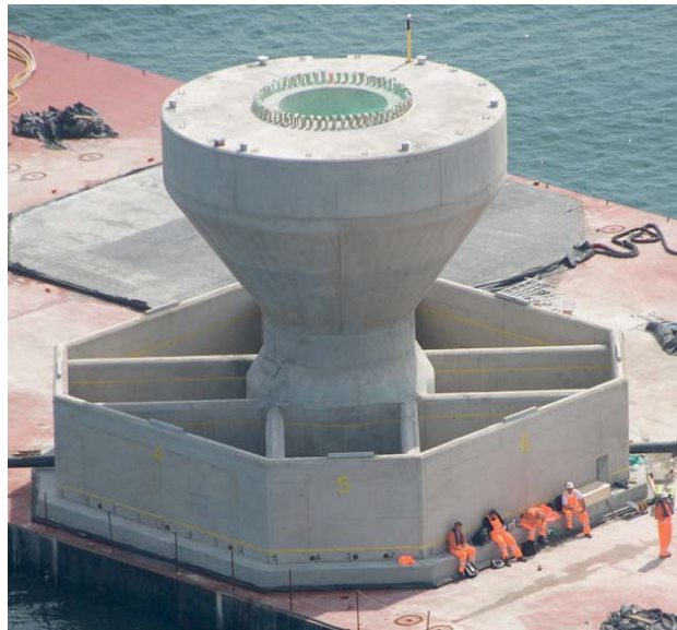
Figure 1.6 Gravity foundation (from www.no-tiree-array.org.uk )
