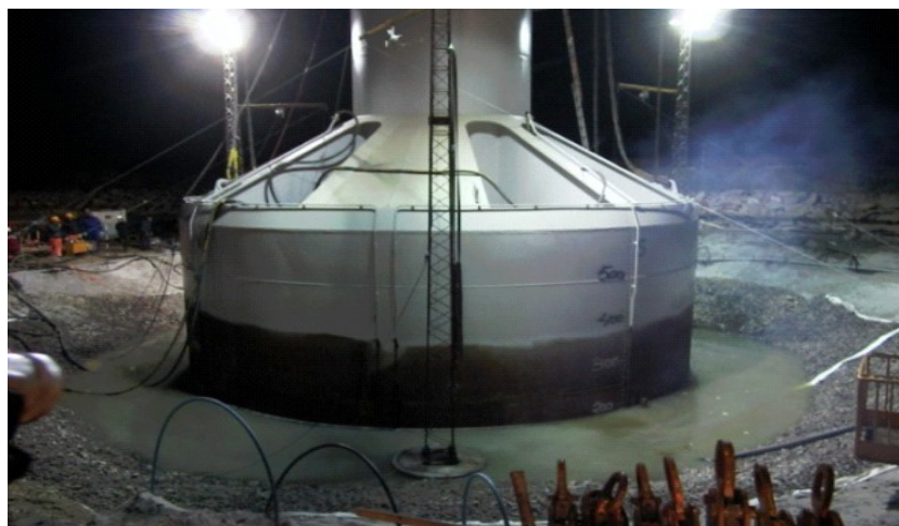
Figure 1.8 Bucket foundation for 3 MW test turbine at Frederikshavn, Denmark (Larsen 2012)
