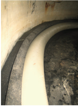
FIGURE 5. INFLATED FIRE HOSE PRESSURING THE MEMBRANE AGAINST THE PILE WALL.
