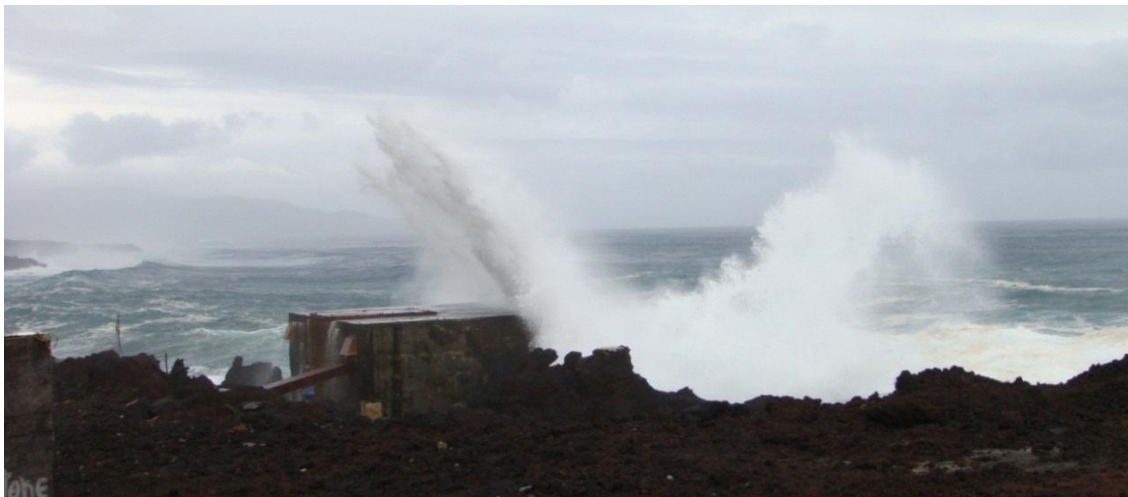
Figure 9: Illustration of a Phase 4 WEC device, the full-scale operational wave energy plant Pico OWC in storm conditions [23].
