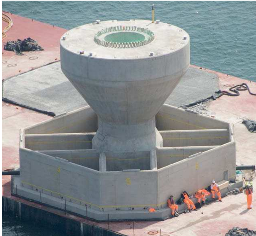
Figure 2: Gravity based foundation to be used as foundation at the Nysted Offshore Wind Farm. The gravity based foundation has been designed with a downward breaking ice cone. www.no-tiree-array.org.uk .
