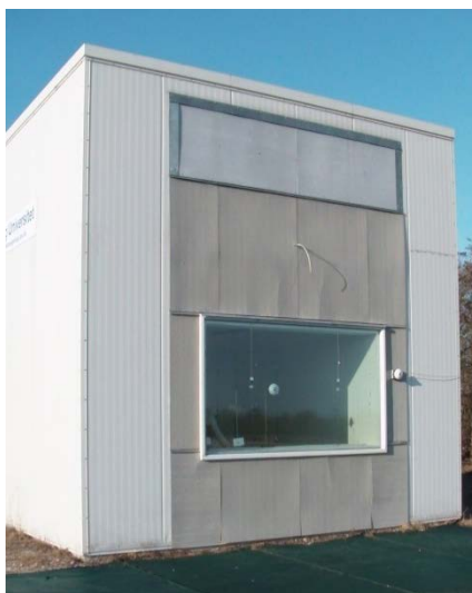
Figure 24: Southern facade of "The Cube".
