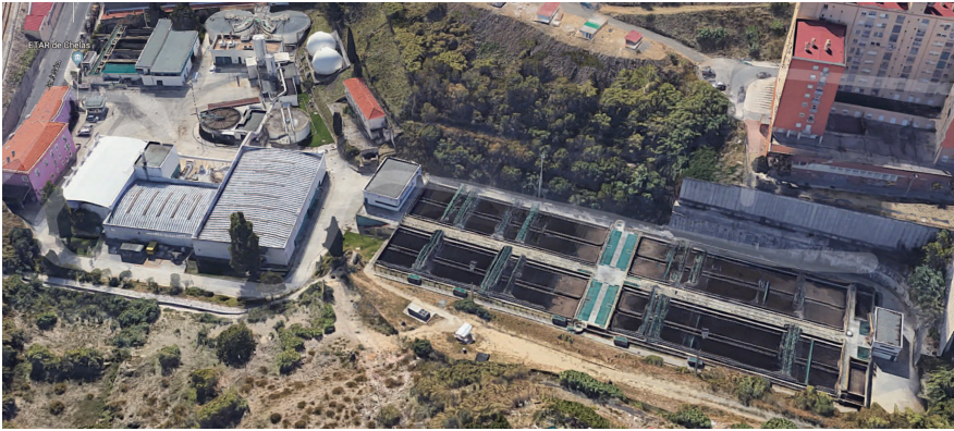
Figure 4.7 Aerial view of the Chelas WRRF.
