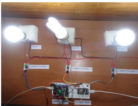
Figure 6. Hardware Implementation of the Power Consumption Monitoring System using IoT
