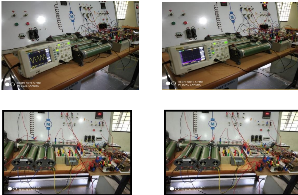
Fig. 3. Hardware Implementation of Wind and solar based Smart Grid
