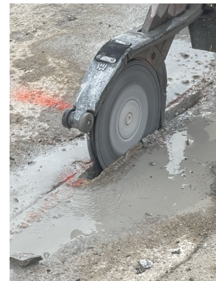
(c) Shear key-way being saw-cut (D3)
