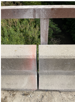
(a) Parapet after saw-cut (D1)
