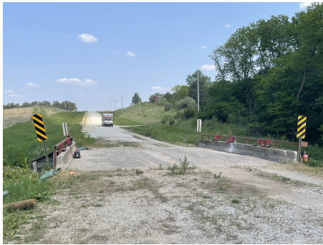
(a) Overview of the bridge including parapets
