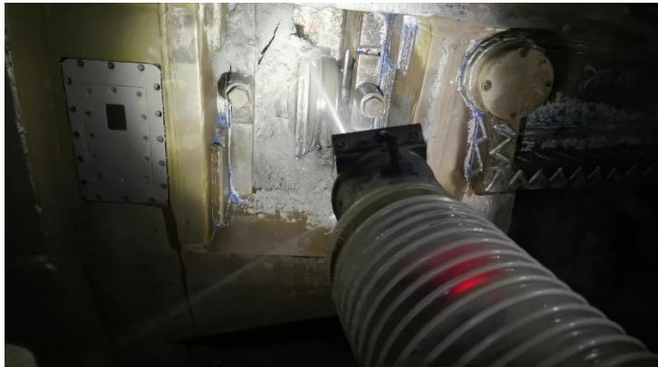
Fig. 18 The snake robot performing cutter cleaning at the tunneling site
