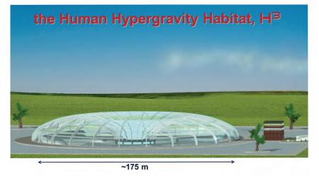
**Figure 11.2** View of the outside structure that accommodates the envisaged human hypergravity habitat ( $H^3$ ). The  $H^3$  is a large-diameter ( $\sim 175$  m) ground-based centrifuge where subjects can be exposed to higher *g*-levels for periods up to weeks or months. The  $H^3$  can be used in preparation for future human exploration programs as well as for regular human physiology research and applications [26, 27]. (*Image* © BERTE byba/van Loon et al. 2012).
