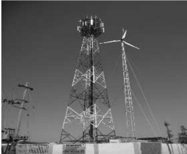
Figure 4 Solar-wind hybrid system at Cellular BTS site Shivarampura, Tumkur, Karnataka, India.
