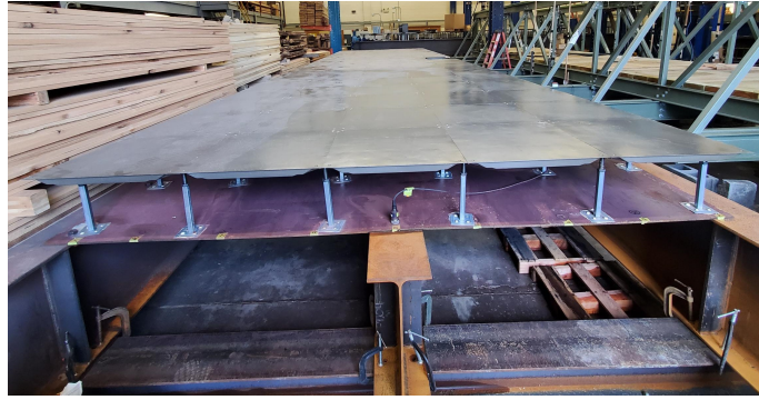
Fig. 2 View of the test specimen with W24x68 beams, a 3/8 in. thick plate, and raised access floor (RAF) on top.
