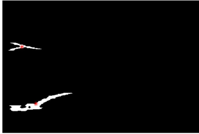
Fig. 11 Binary image of the detected cracks on a sample after the edge masking and morphological filters are applied. The centroids of the detected cracks are calculated and shown as red stars.
