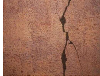
Figure 2.2 :Noise-polluted pipe wall
