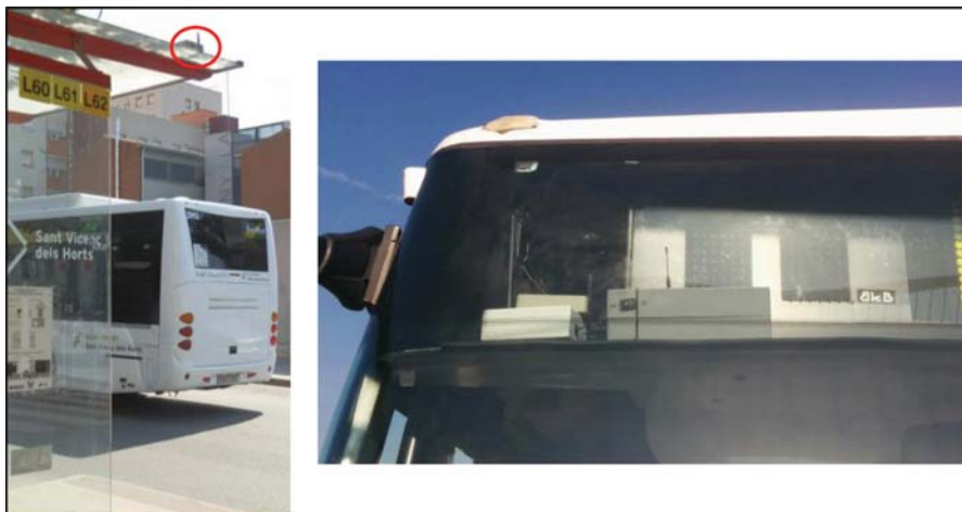
Figure 7.11 Delay Tolerant Network devices. Bus passing close to a low-power wake-up sensor device installed in a bus stop. Detail of the equipment (gateway) installed in the bus.
